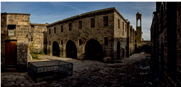
After restoration in 2014
