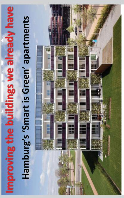
passive house 'plus' ... PV modules in balcony balustrades ... solar thermal roof units ... climbing plants/solar shade ... PCM curtains and thermal store ... heat pumps.
